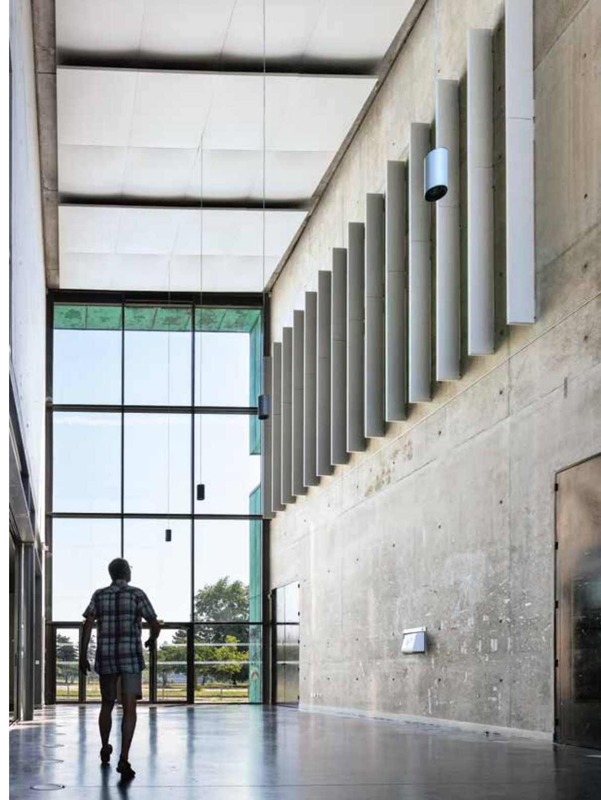
Single-sided Stereo panels cladding a ceiling and double-sided panels used against a wall. Pessac, Maison des Arts, Bordeaux Montaigne University, arch. Massimiliano Fuksas, 1994. Rehabilitation: Poggi Architecture, 2013.
