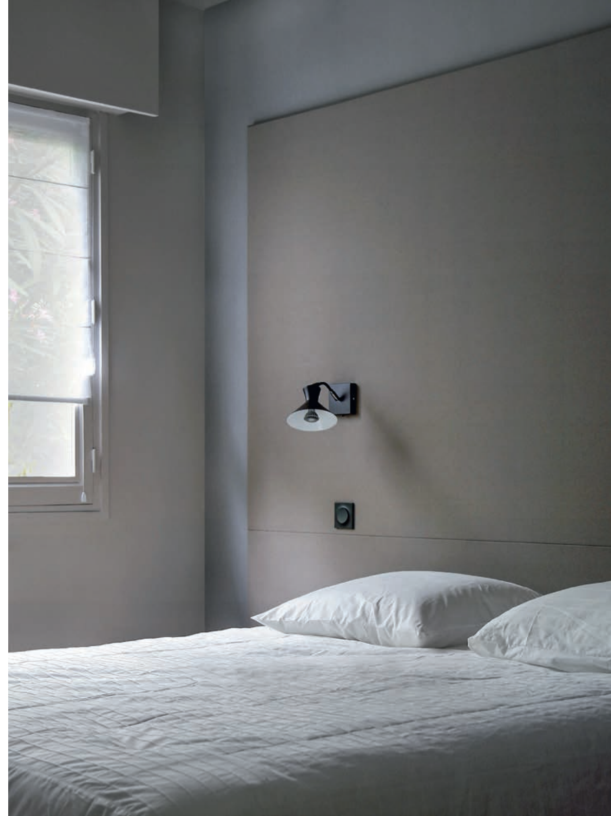
Vibrasto 30 mm fitted as a panel, private home, Bordeaux (renovation), 2017, arch. Christine Bernos.
