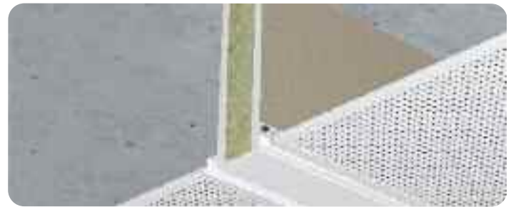
Finishing recess under sound barrier for receiving removable partition.
