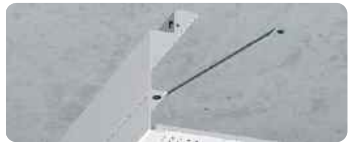
Tall two-part drop with additional support.
